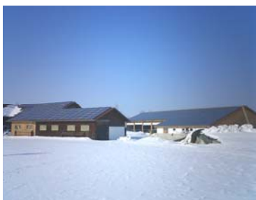
Sun-Earth brand solar modules installed at mountain with altitude more than 5000M.
